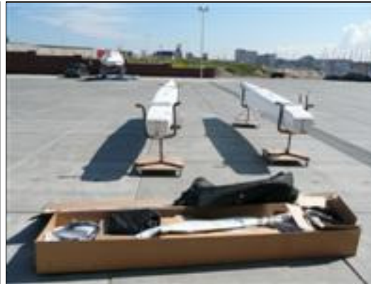
Mounting the beams Step 1 & 2
